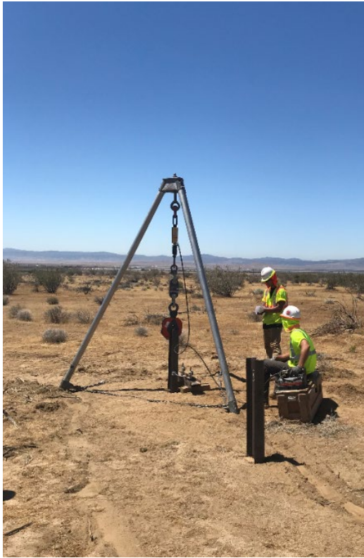
Figure 5: Axial Load Testing
