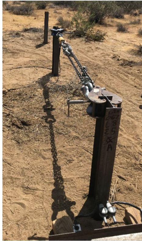
Figure 6: Lateral Load Testing
