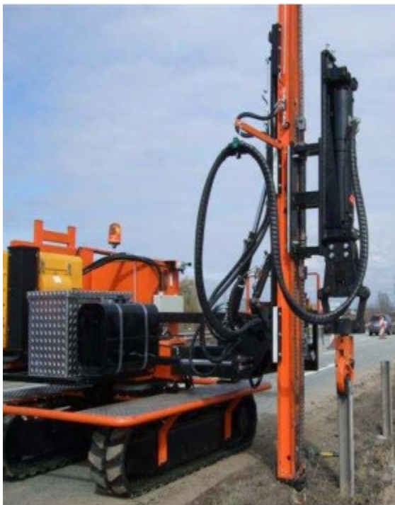
Figure 4: Example Hydraulic Hammer Rig
