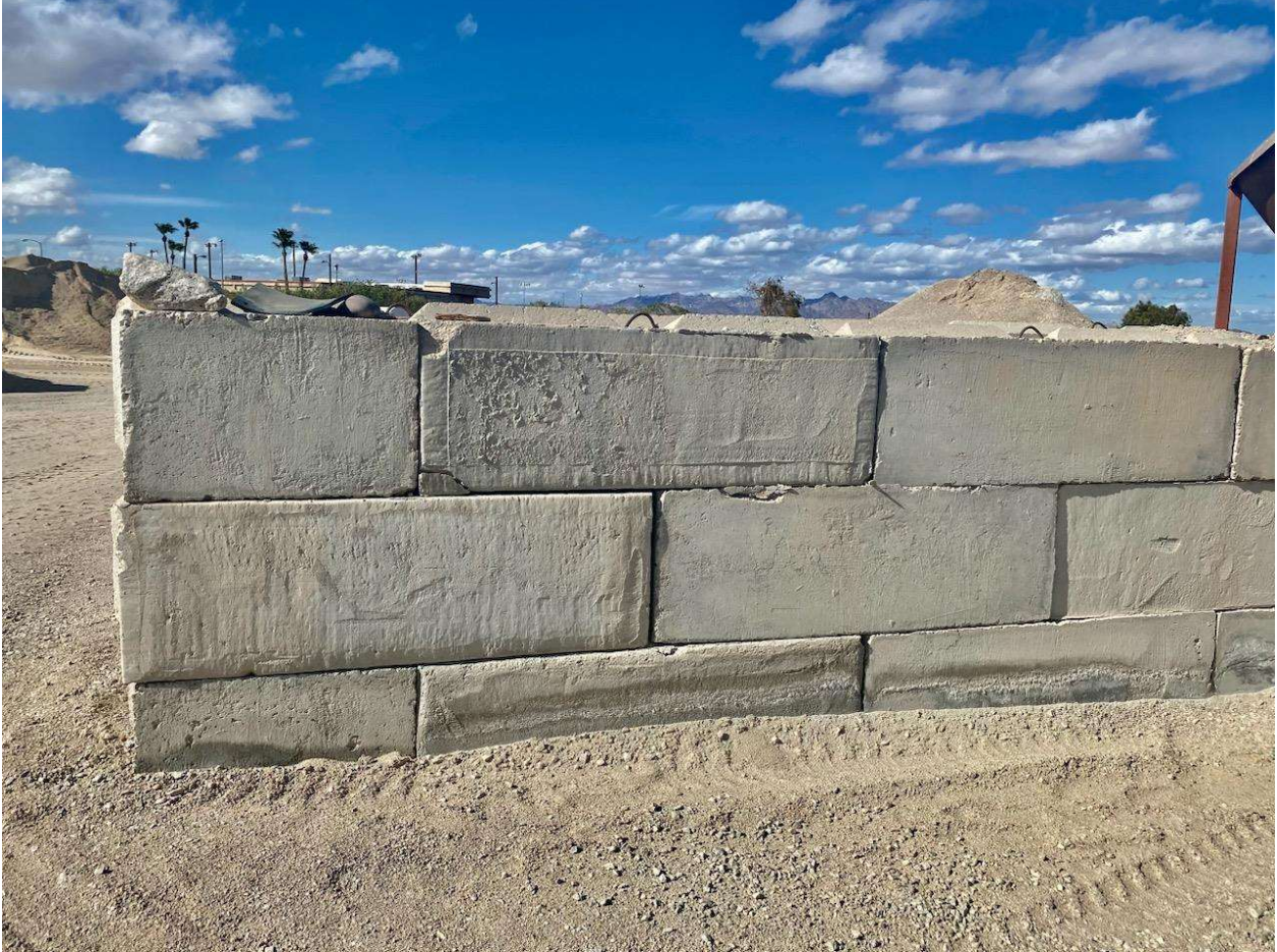
Figure 3. Concrete Blocks for Chain Connection.
